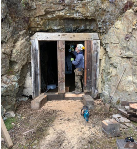
Figure 4 - New heavy timber frame.
