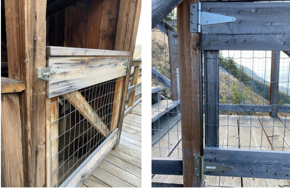
Figures 11&12 – new hinges and latches on gates that had been ripped off their mooring
