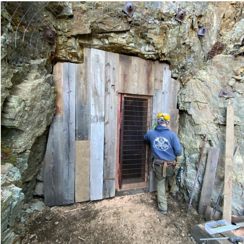
Figure 6 – New Portal Number 1 with 3" plank cladding.
